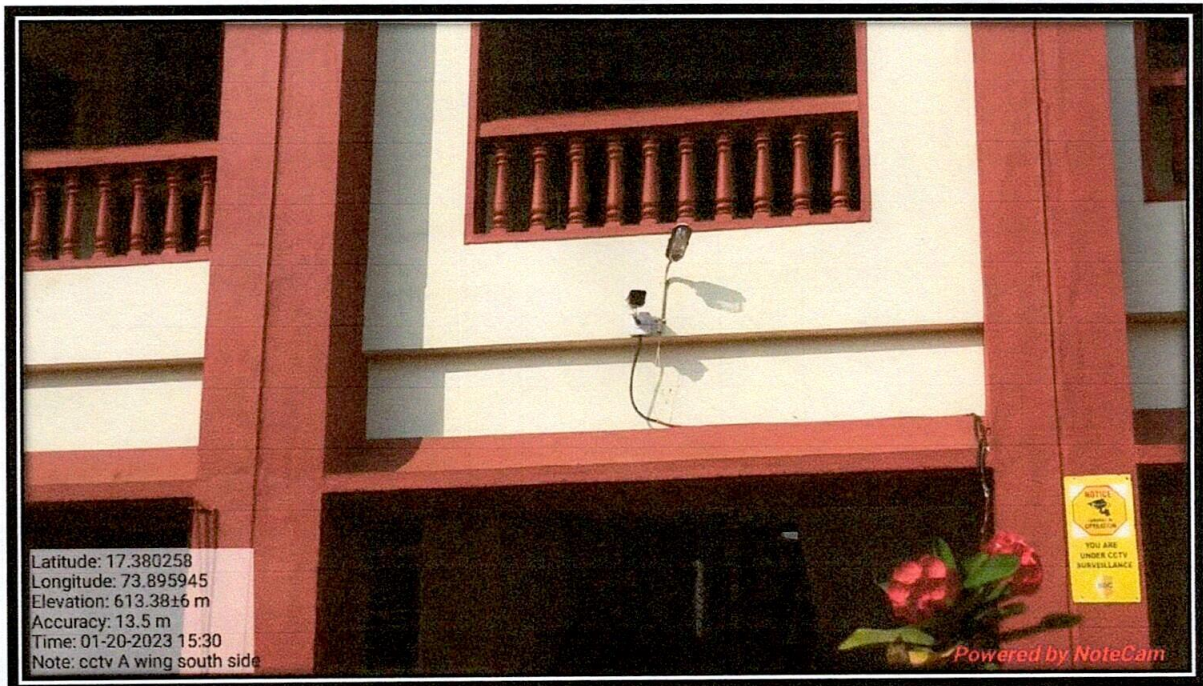
A WING FIRST FLOOR SOUTH SIDE:-
